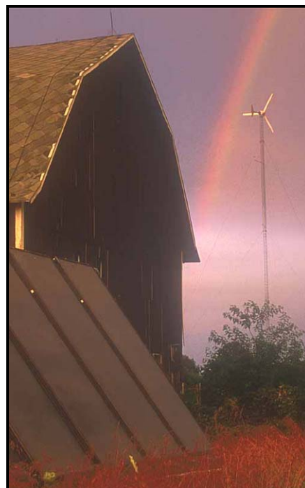
Solar panels & wind turbine at Inn Serendipity (JOHN IVANKO/ecopreneuring.biz and ruralrenaissance.org)
